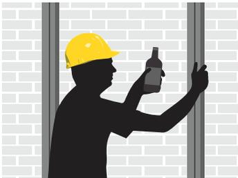
Thoroughly clean oil surface of loose debris. Wipe the joint surfaces and remove dirt & contaminants. Allow the surface to dry. Samrat recommends Dow Corning R40 Universal Cleaner or R41 cleaner Plus.
